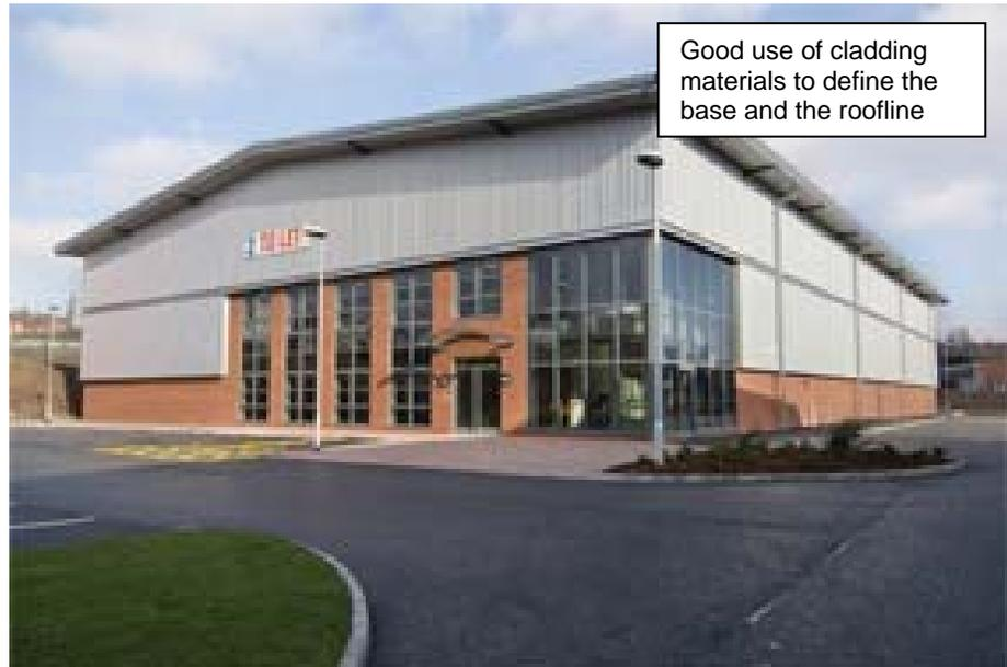
4.3.7.2 The ideal ratio for defining the base height is 4:1. For example, if the building height is 12'-0" the base should be 3'-0".
