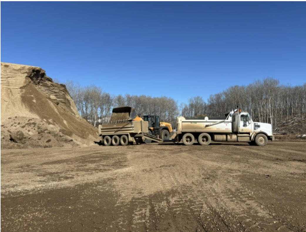
PW 0.11 Pushing up Gravel at the Hwy 53 Pile
