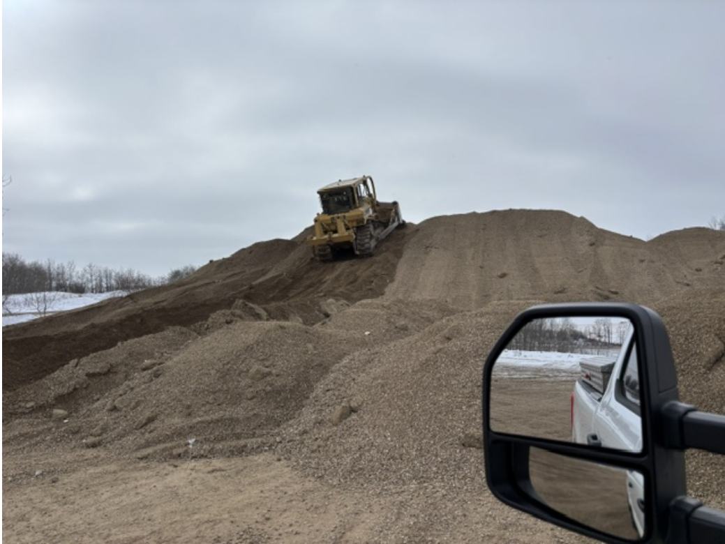
PW 0.10 Pushing up Gravel at the Hwy 53 Pile
