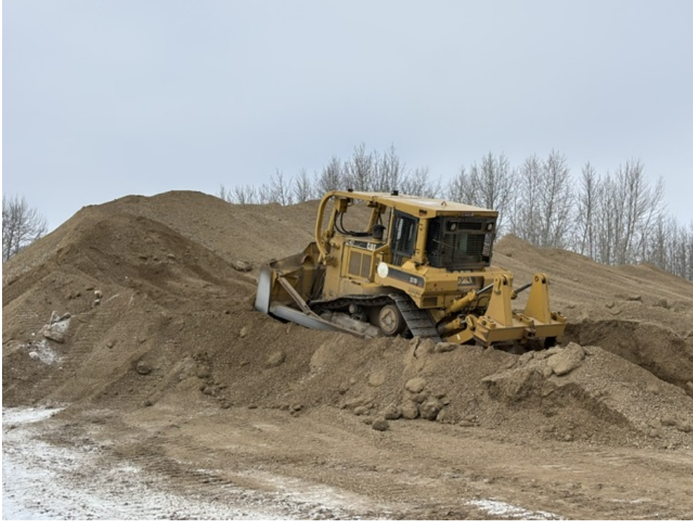
PW 0.07 Pushing up Gravel at the Hwy 53 Pile
