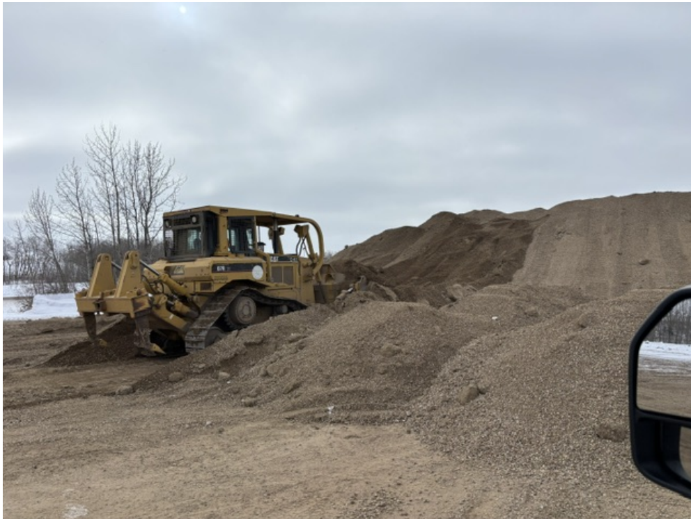
PW 0.08 Pushing up Gravel at the Hwy 53 Pile
