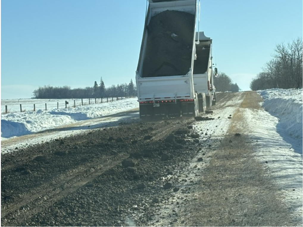
PW 0.12 Patching TWP Road 38-0
