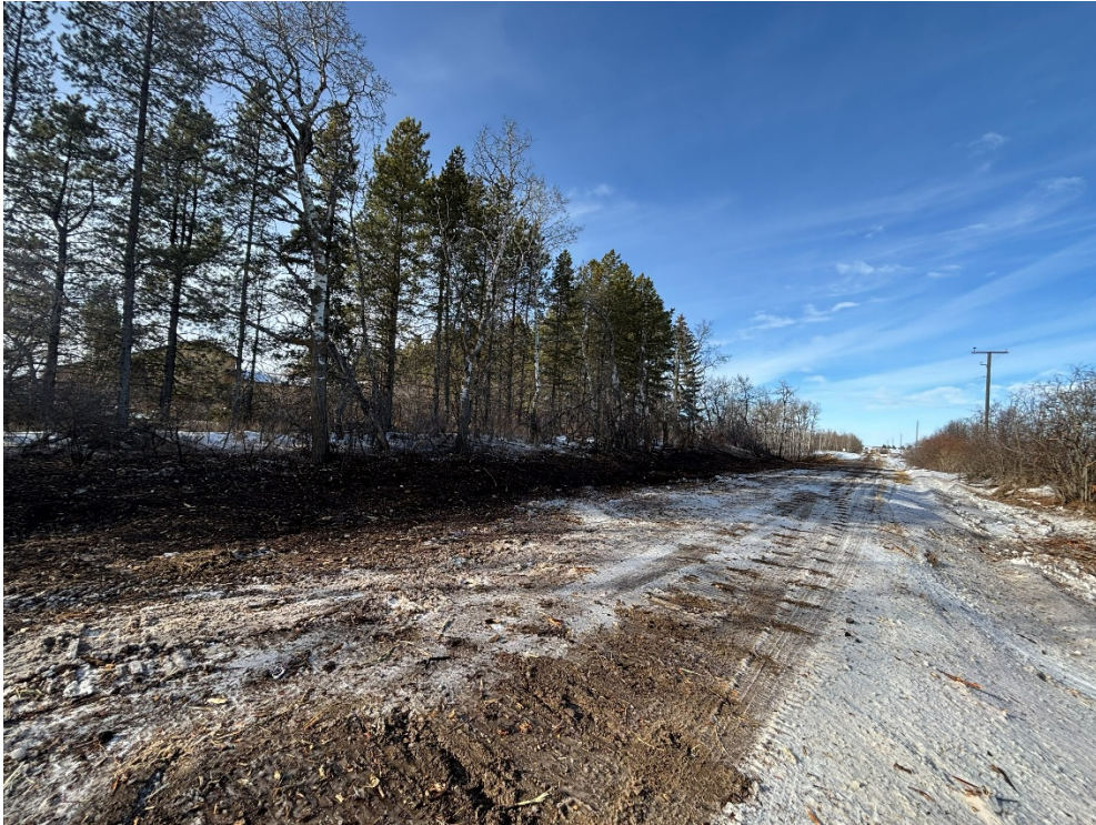
PW 0.03 Range Road 21-2 South of Hwy 601 Brushing
