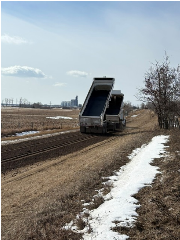
PW 0.13 Patching TWP Road 39-0 East of Hwy 835
