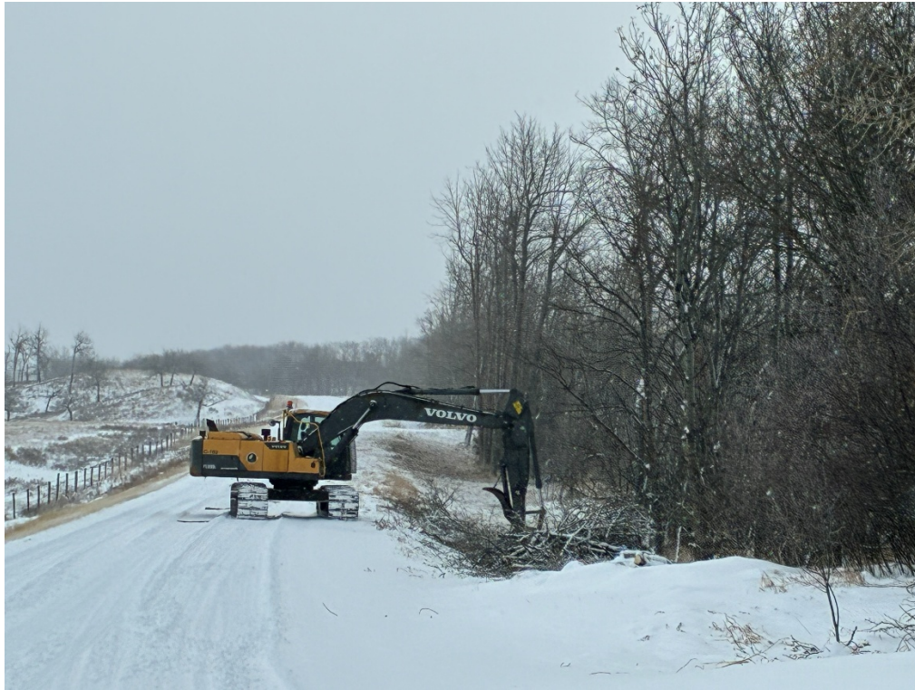
PW 0.05 Chainsaw Crew/Trackhoe Mulcher TWP Road 37-2 West of Hwy 835
