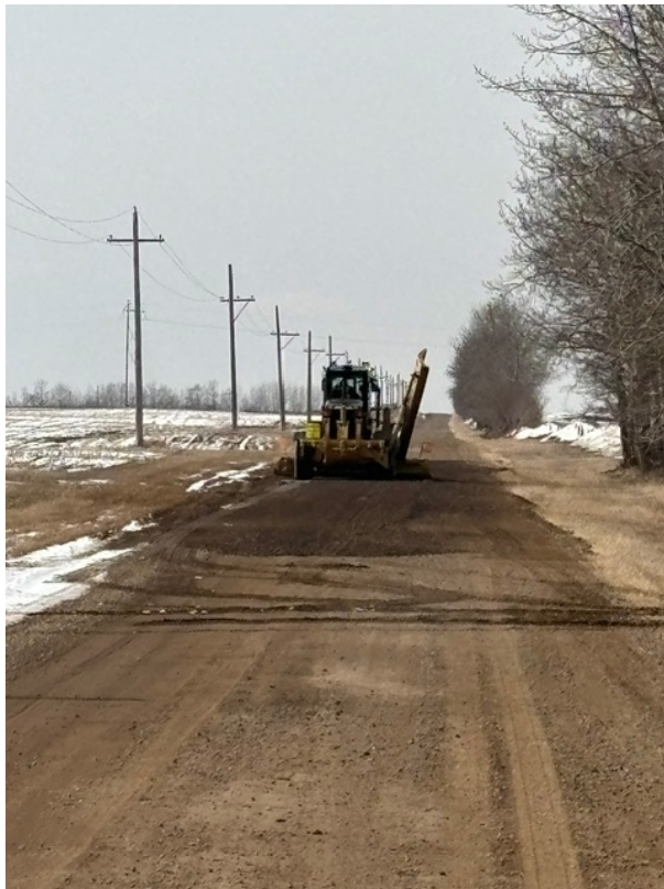
PW 0.15 Grading Gravel Patch Spots
