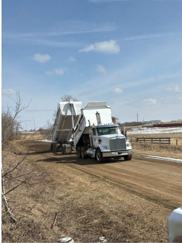
PW 0.14 Patching TWP Road 39-0 East of Hwy 835
