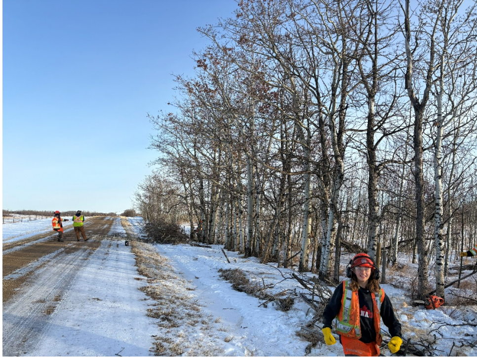
PW Figure 0.06. Chainsaw Brushing
