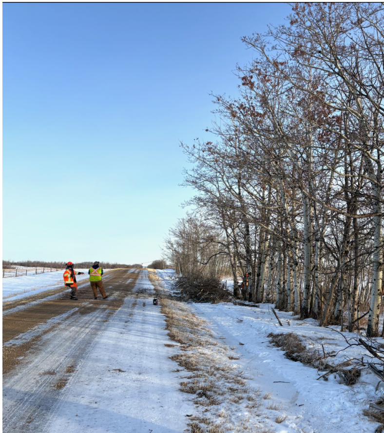
PW Figure 0.07. Chainsaw Brushing
