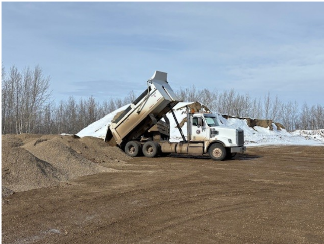
PW Figure 0.15. Working on Hwy 53 Stockpile
