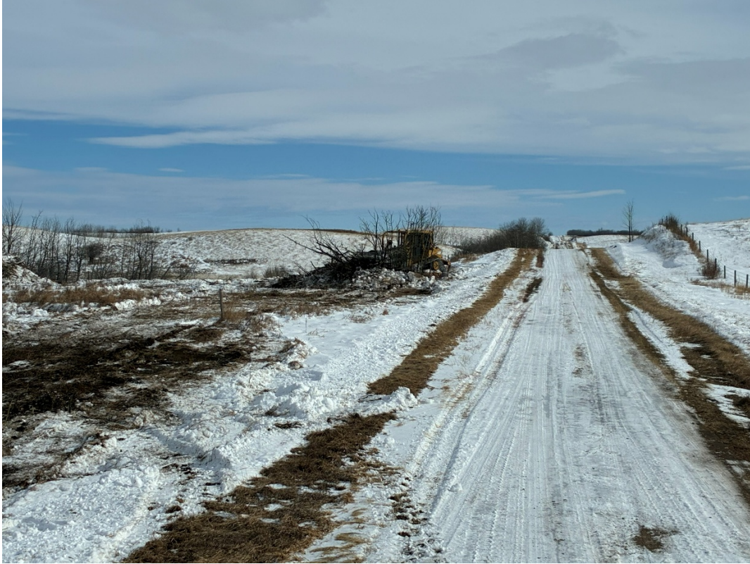
PW Figure 0.08. Dozer Work on Rge Rd 19-1
