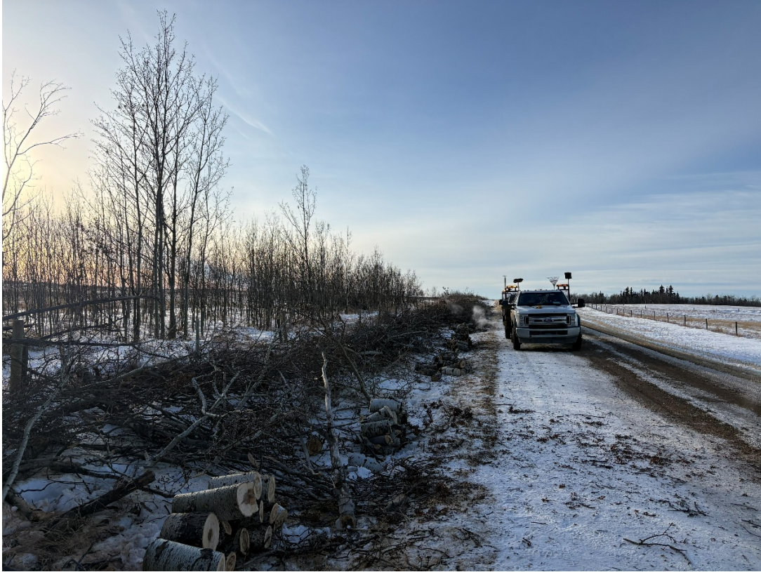
PW Figure 0.04. Chainsaw Brushing
