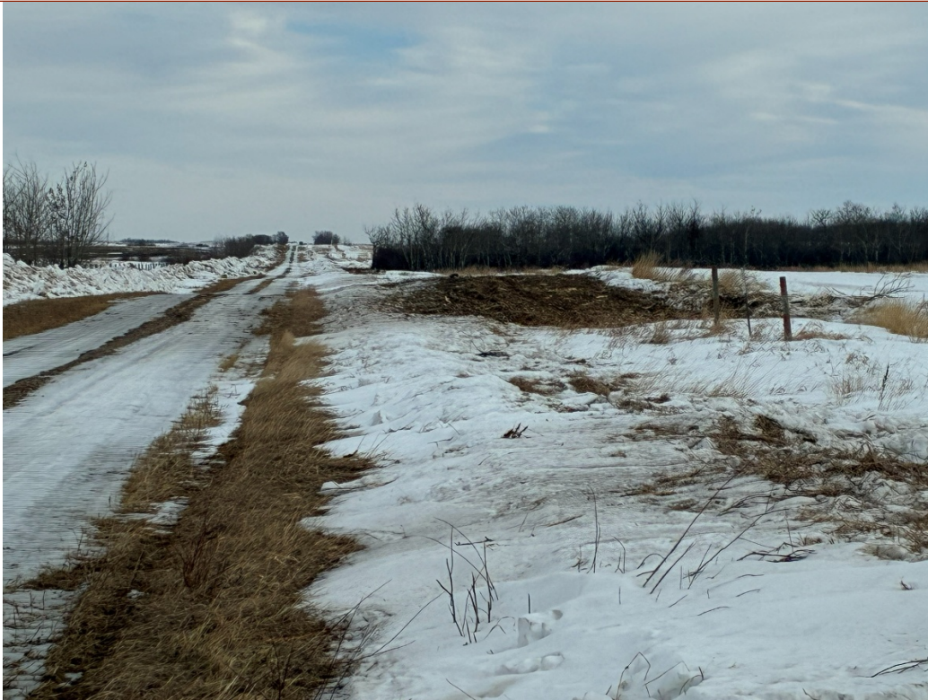
PW Figure 0.01. Rge Rd 17-0 & Twp Rd 38-0 Bobcat Mulcher Along Fenceline
