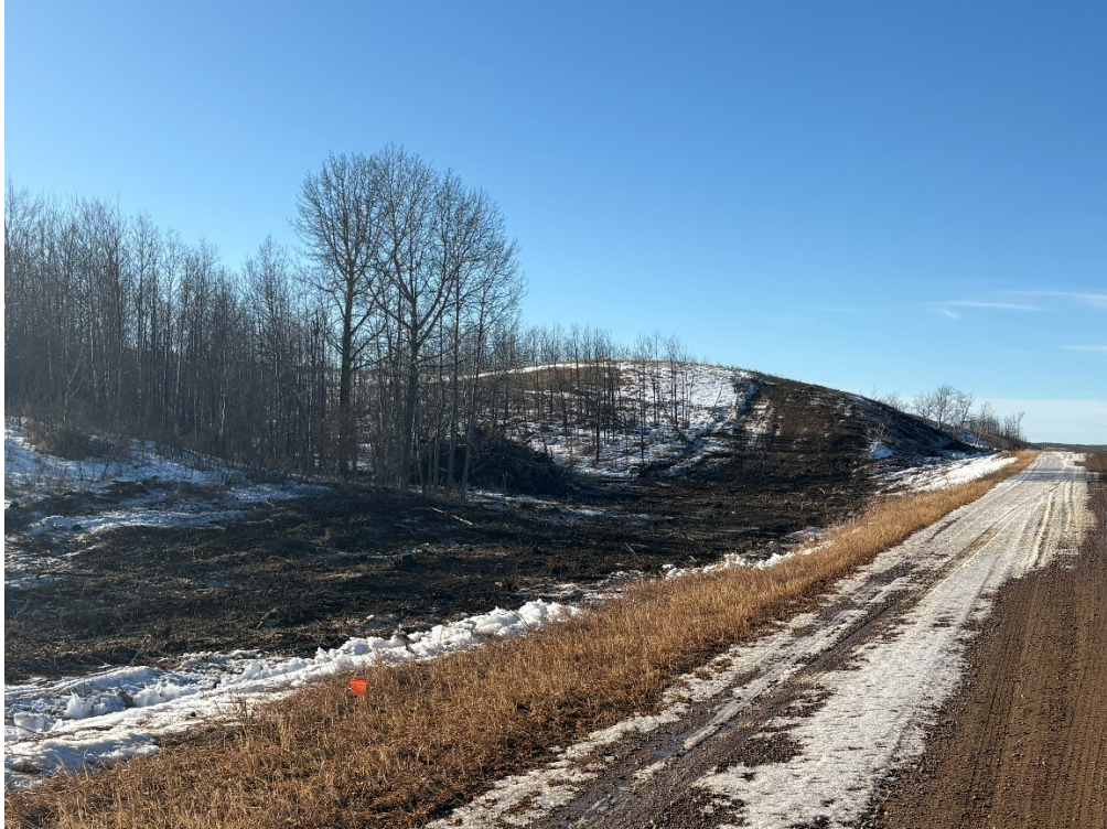
PW Figure 0.10. Dozer Work on Rge Rd 19-1
