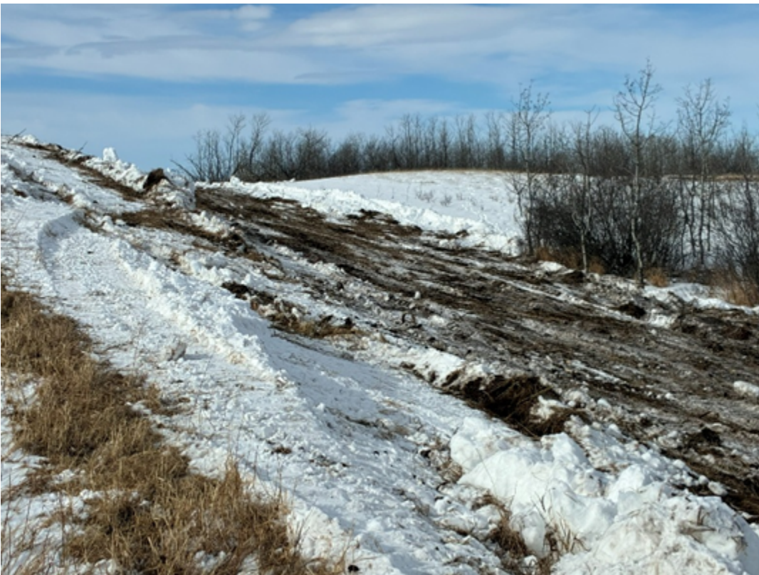
PW Figure 0.09. Dozer Work on Rge Rd 19-1
