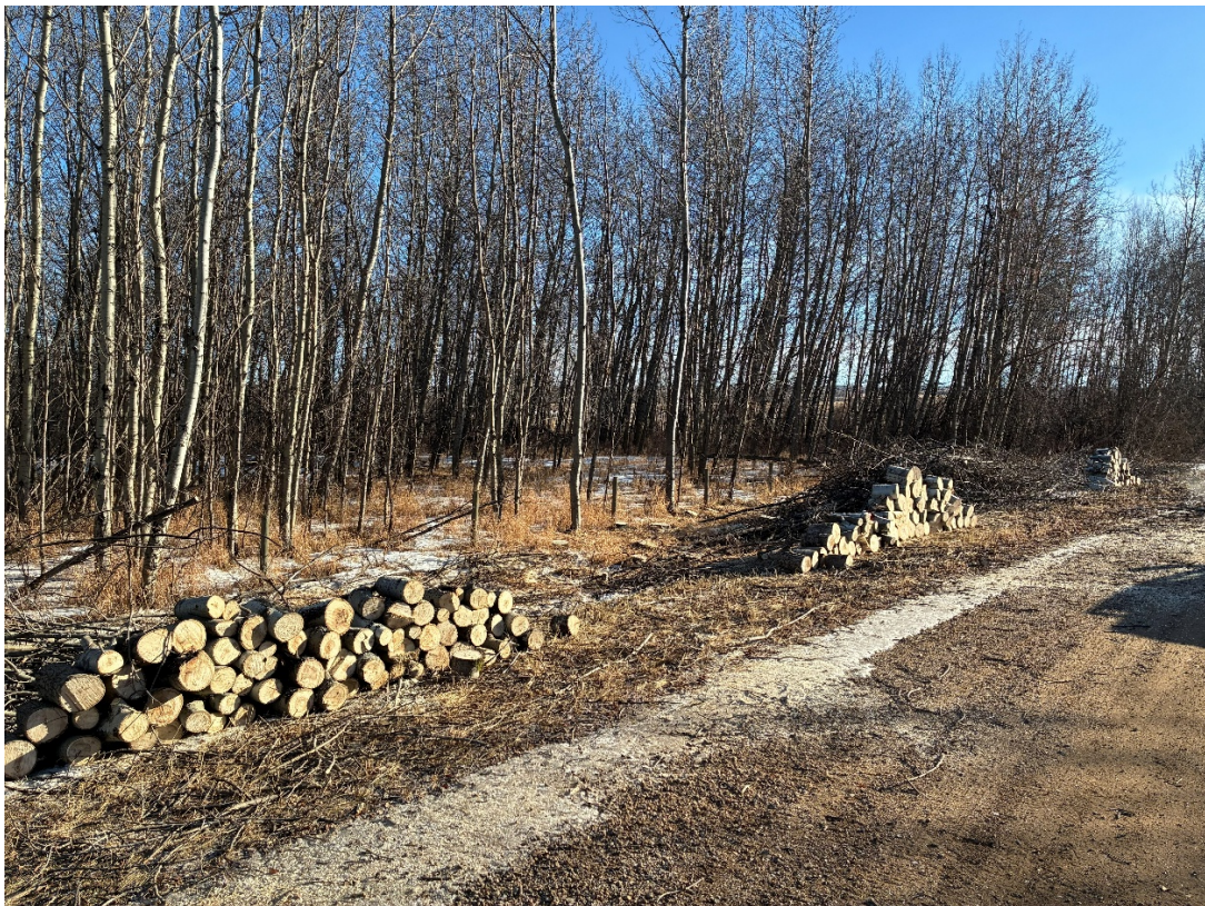
PW Figure 0.05. Chainsaw Brushing
