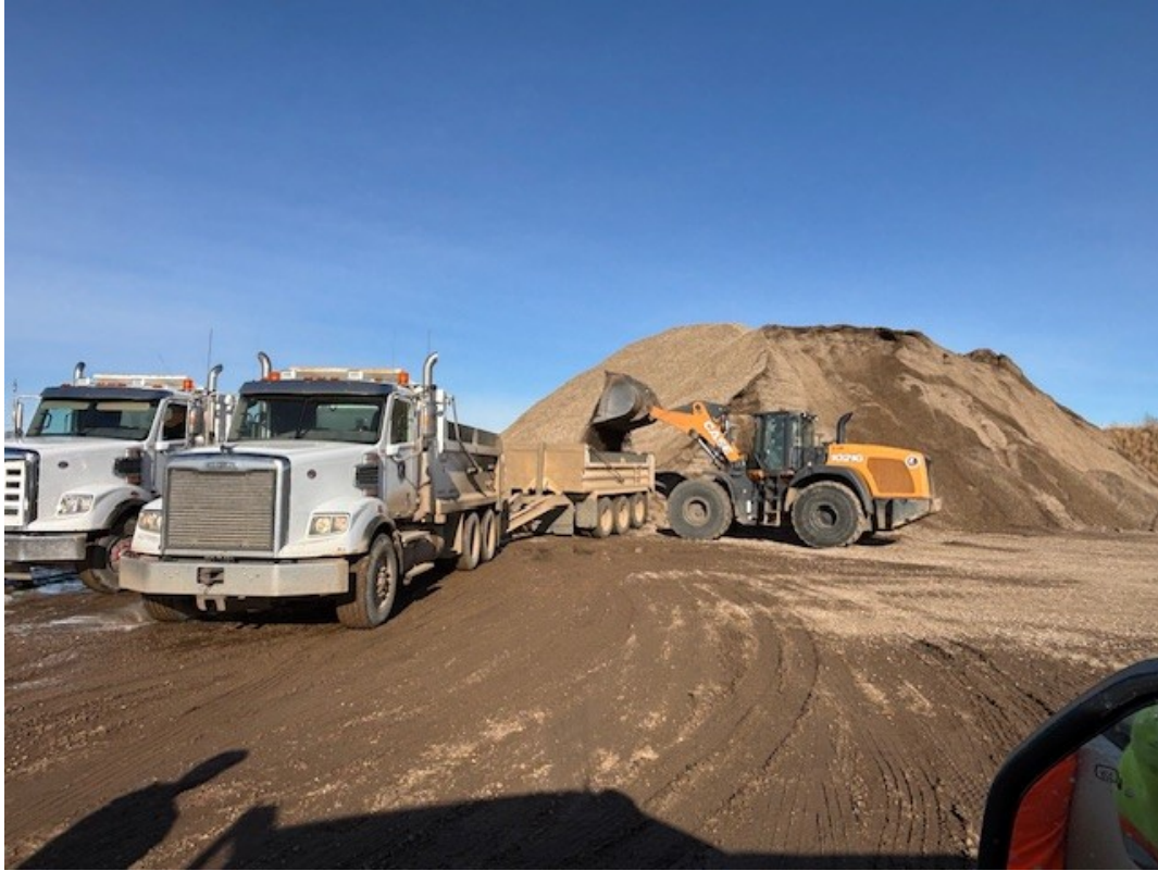
PW Figure 0.16. Loading Trucks at Collins Pit
