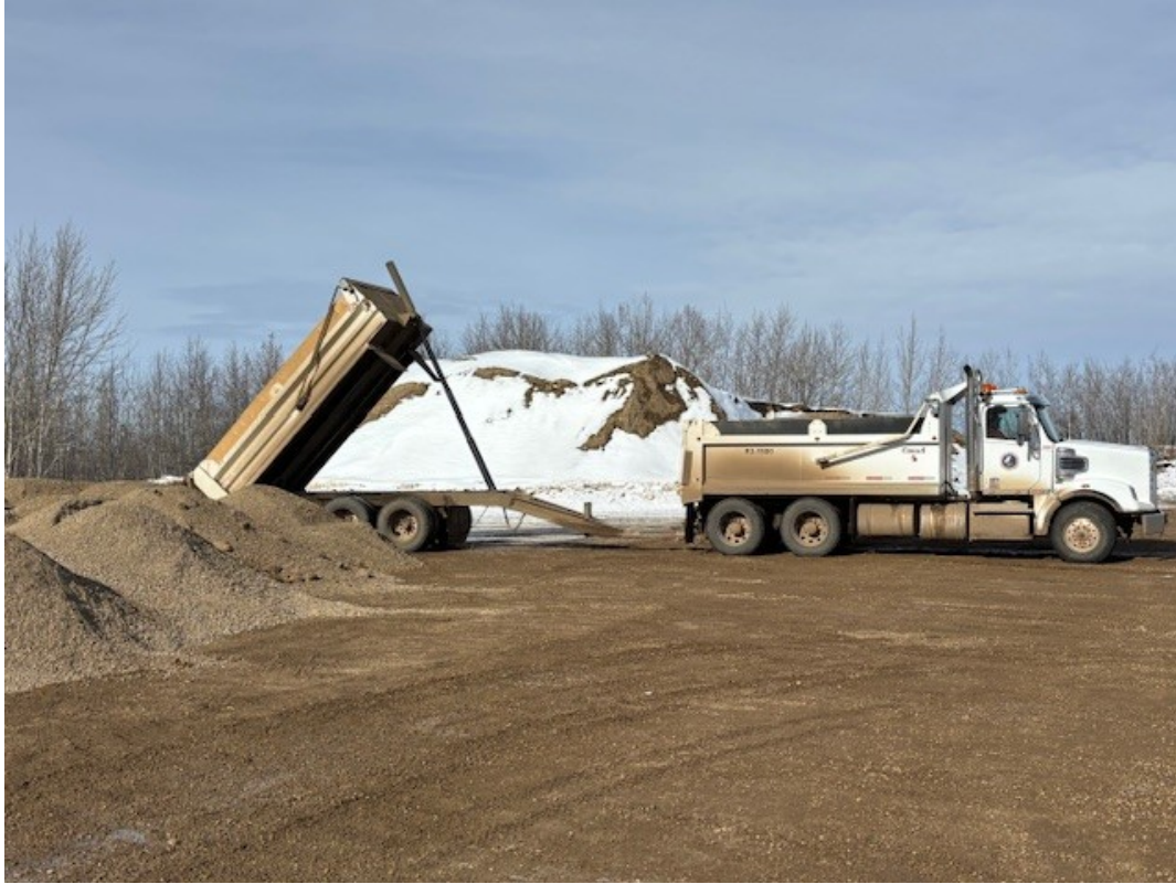
PW Figure 0.14. Working on Hwy 53 Stockpile
