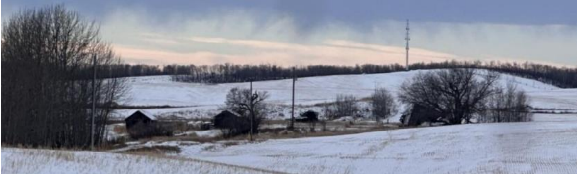
Photo 1: View of the abandoned buildings located on the proposed parcel, looking west
