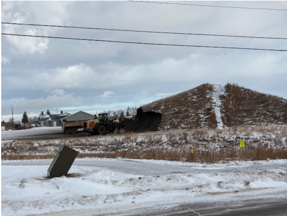
PW 0.10 – Working on Topsoil Pile
