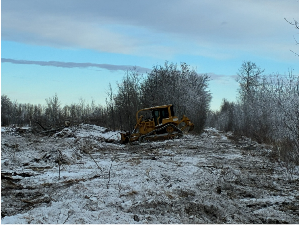
PW 0.01 – Brushing Work
