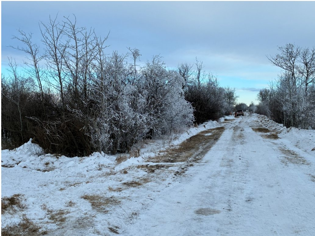
PW 0.04 – Brushing Work
