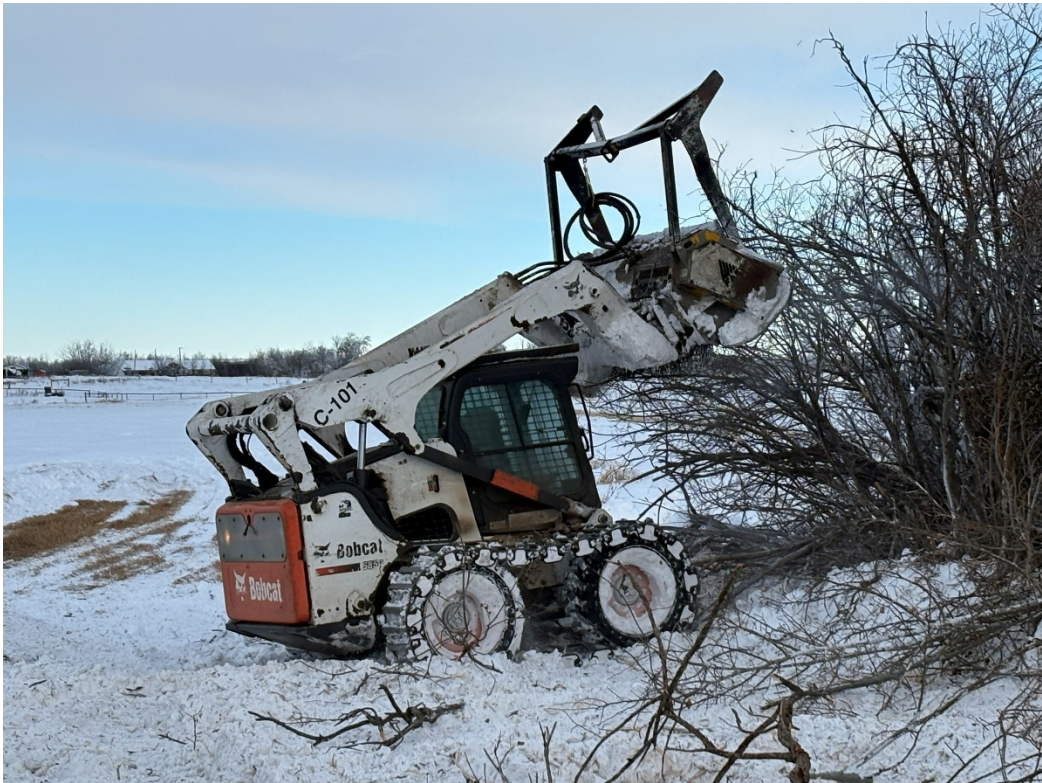
PW 0.02 – Brushing Work
