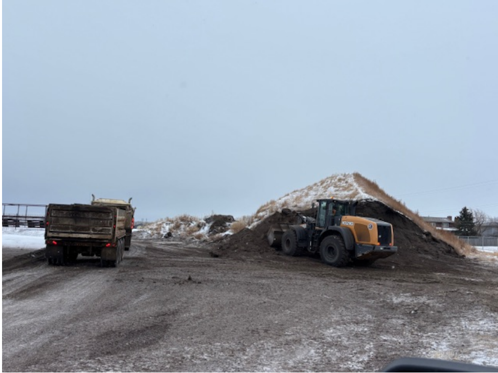
PW 0.09 – Working on Topsoil Pile
