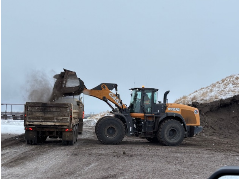
PW 0.11 – Working on Topsoil Pile
