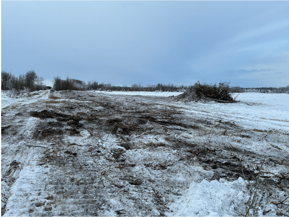
PW 0.03 – Brushing Work
